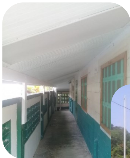
External corridor completed with 4x2 light fixtures installed and finish flush with treated groove ply ceiling, which was also coated with marine paint.
