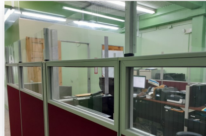
Installation of plexiglass at work stations
